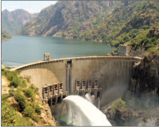
Cahora Bassa, Mozambique. Built in the final stages of Portuguese administration, to export power to Eskom, South Africa, under a PPA defined in Rand, without any provision for exchange rate adjustment or escalation. Shortly after commissioning, the HVDC transmission line was blown up and remained unusable for more than 10 years. By the time the line was reinstated, the Rand had devalued by a factor of ten, and the project was committed to deliver energy at less than US¢1/kWh. The PPA was eventually renegotiated after years of sub-economic operation.
